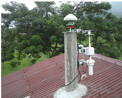
PRS antenna at Bhur RDC, Gelephu
