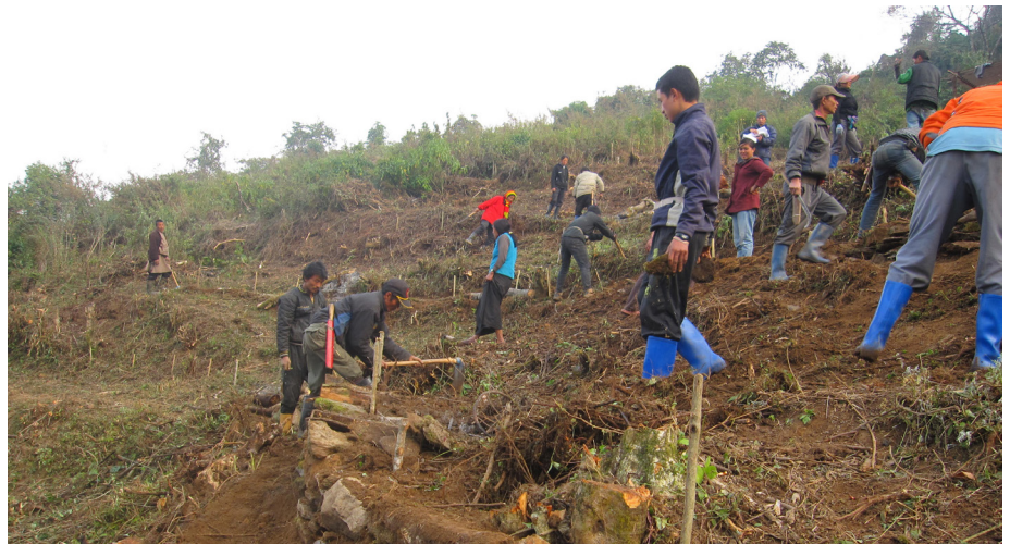
Beneficiaries clearing the land for settlement purpose
