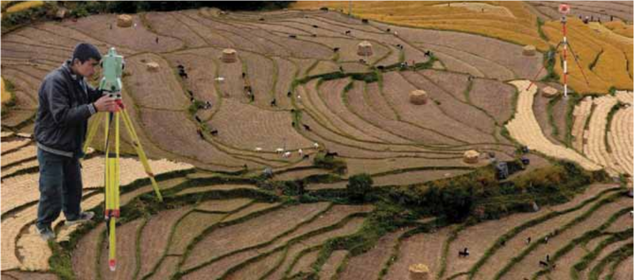
Surveying using Total station
