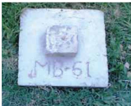
Concrete control point
